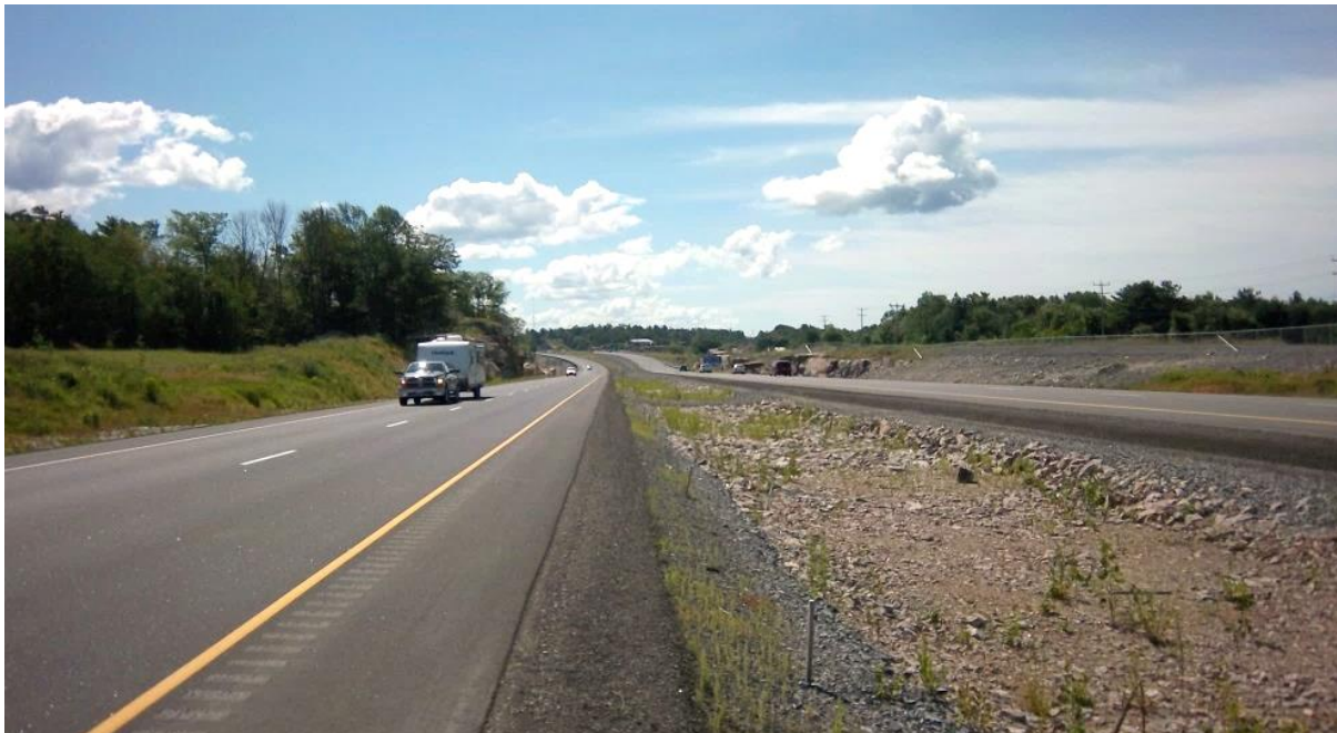
Example of a Four-Laned Section of Highway 11/17
